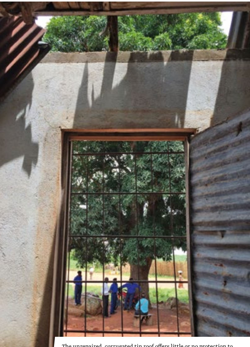
The unrepaired, corrugated tin roof offers little or no protection to the weapons or ammunition against either theft or the elements.
