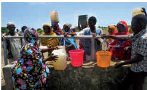
A water filtration plant set up under UNDP's Community Security and Arms Control programme in White Nile State, Sudan, June 2013.
